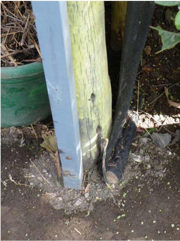
Fig. 3 Bottom of screening (rolled around pole) to be buried for a biocontrol agent mass-rearing structure, to prevent entry of insect predators from outside and exit of insects to be mass-reared inside the structure at the soil-screening interface.
