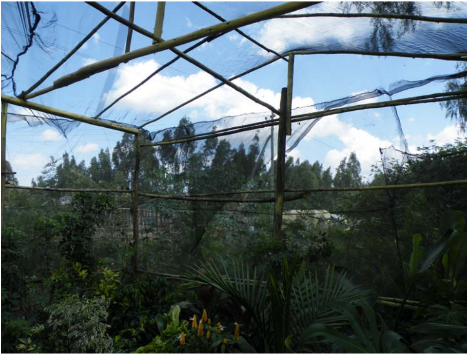
Figure 1a & b: Greenhouse structure (note that a biocontrol agent mass-rearing structure should be lower in height than the structure shown in photo, to enable easier collection of insects from ceiling) used by nursery industry en route from Addis Ababa to Sodore. It is recommended that a similar design is followed for parthenium biocontrol mass-rearing structures.
