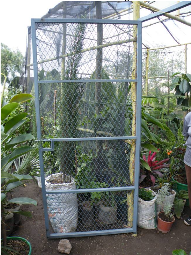
Fig. 4 Lockable gate (will need fine screening on gate for biocontrol agent mass-rearing structures)
